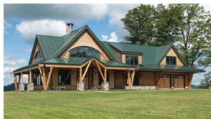
Post and Beam (Timber Frame)
